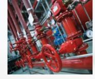
In sprinkler plants large quantities of water have to be distributed under high pressure through thick pipe strings. This is where three types of Götze valve fittings are applied, ensuring a perfect functioning: Pressure reducers regulate the water distribution. Safety valves let off excessive pressure. And overflow valves ensure a smooth pump operation.
